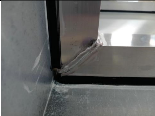
8. The reinforcement in the middle were welding from 3 sides, the welding was done with gap
